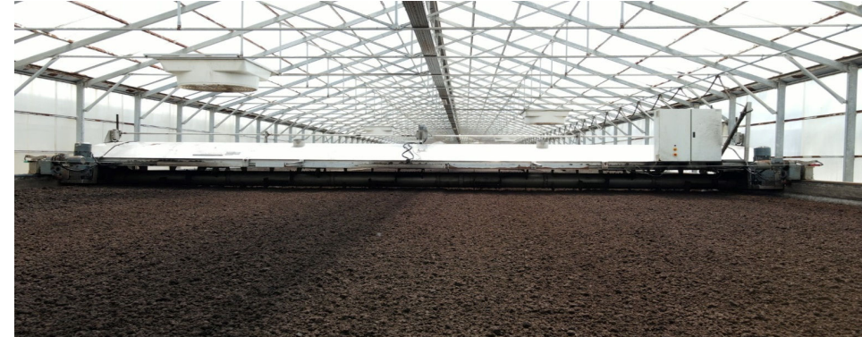
İZBAŞ FREE ZONE WWTP, TURKEY
